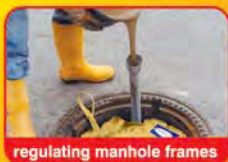
regulating manhole frames
