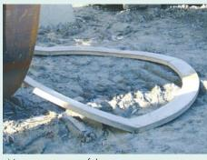
a) Improper support of the pressure transmission devices
