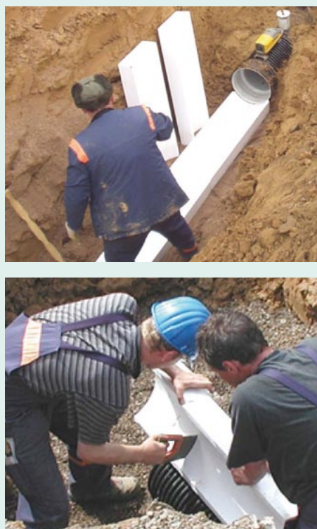
Figure 11 Practical application of bedding cushions: laying (top left), cutting to size on site (bottom left), complete encapsulation as a variant (right)
