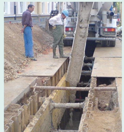
Figure 8 Installation of flowable self-compacting filling materials in narrow trench width
