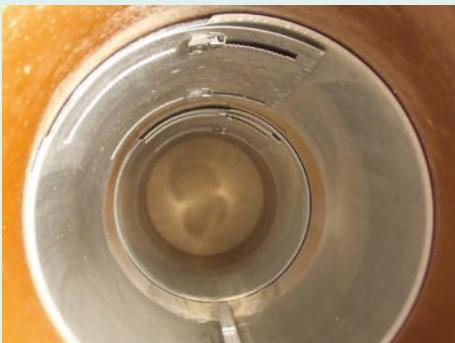
Example of sleeve without (top) and with (down) visible traces of high-pressure flushing
