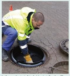
In the practice test: A technician installs odour-filters in manholes on the IKT compound
