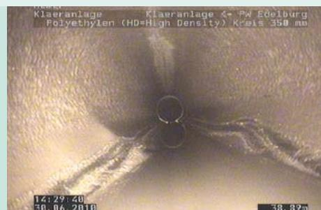
Deformation caused by point load in an HDPE pressure waste-water conduit
