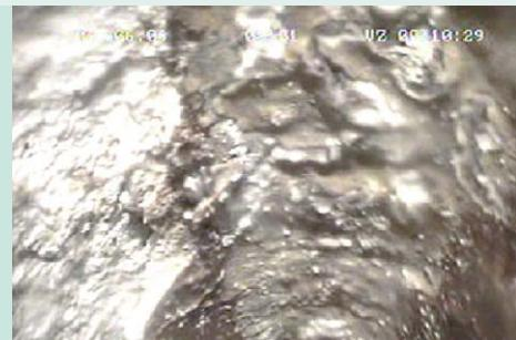
Detachment of material on the pipe wall of an asbestos-cement drinking-water conduit
