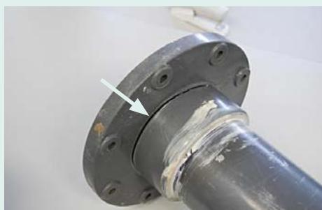
Cracking at a flanged joint in a PVC pressure waste-water pipe at the pumping station
