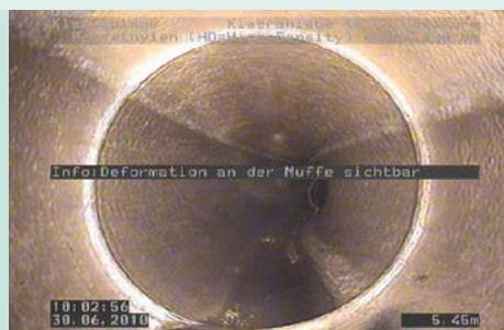
Ovality caused by point load in an HDPE pressure waste-water conduit
