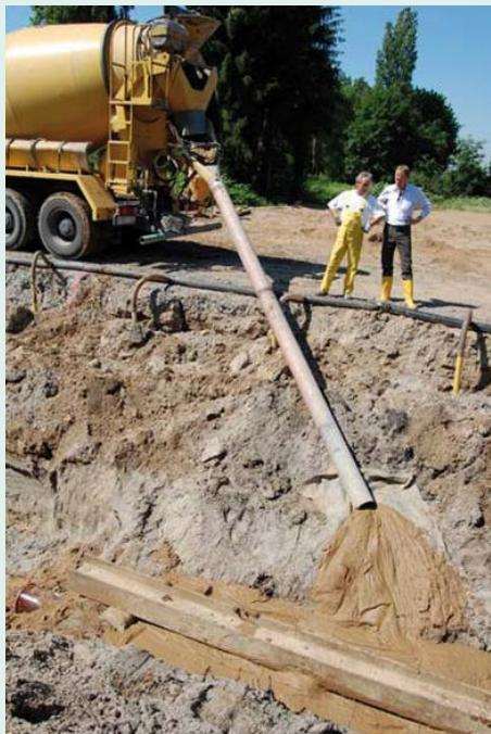
Function: in-fill material for drain/sewer and conduit engineering
