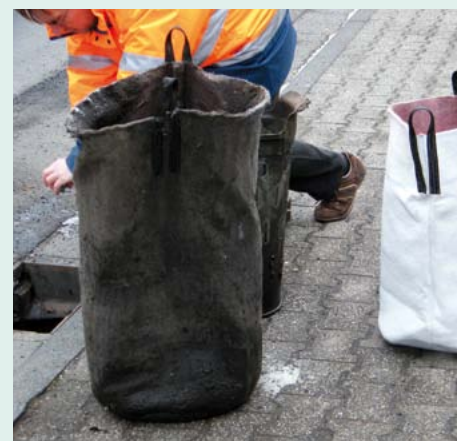
Inspection of a road gully equipped with a geotextile filter bag
