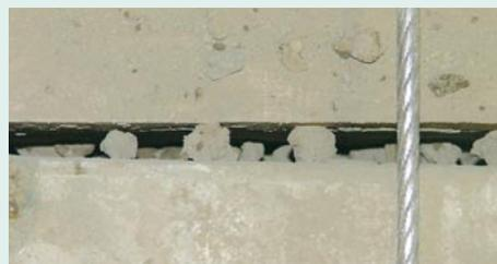
b) Dirt of a gaping joint in the sole area
