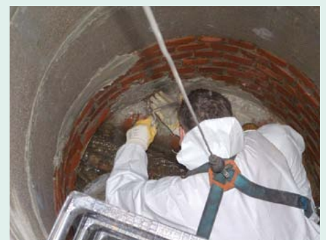
Sealing work in practice: cementitious waterproof plugging compound
