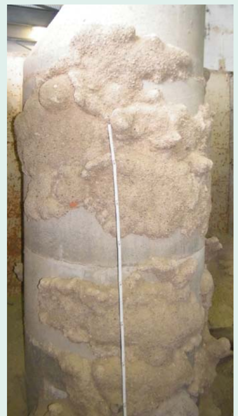
Polyurethane injection body on the exterior of a manhole
