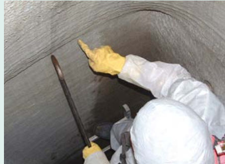
Acceptance inspection: visual assessment of the coating
