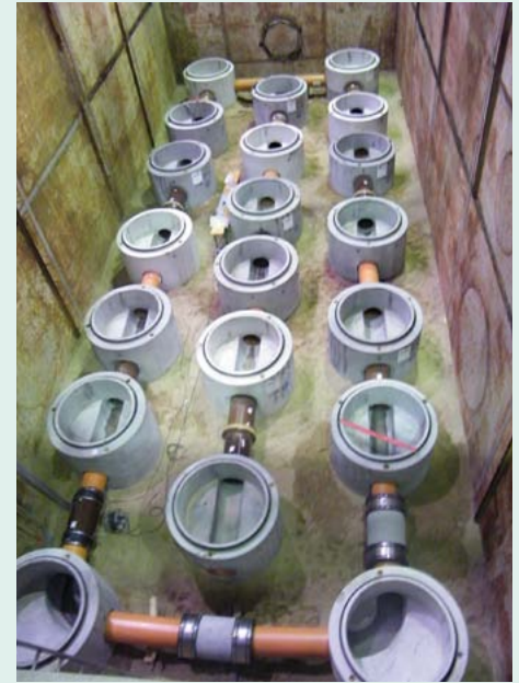
Installation of the manholes in the large-scale test facility
