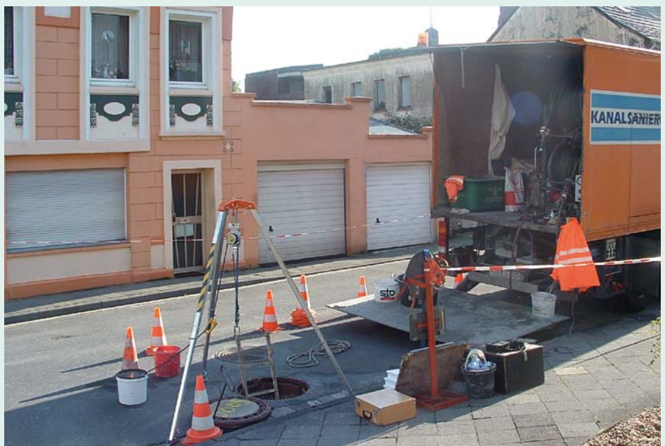
Manhole renovation in practice
