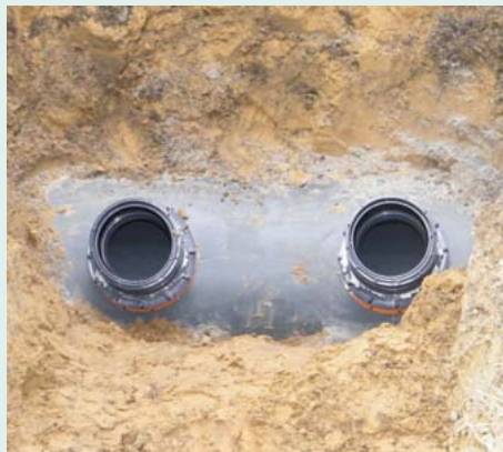
Connex connection following installation (from site study)
