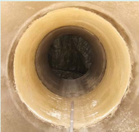
Figure 1: Repair methods in IKT projects: short-liners
