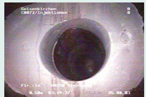
Figure 3: Repair methods in IKT projects: Injection/pressure refurbishing on sewer laterals
