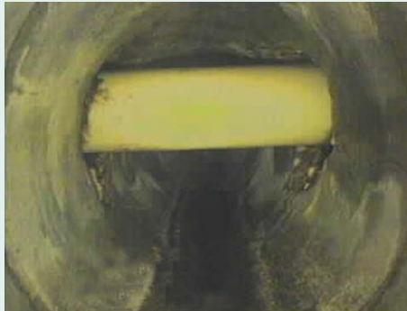
Figure 4: Piercing techniques piercing other pipelines
