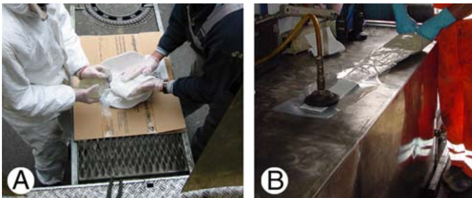
Figure 7. Top hat liner resin impregnation A Only manual resin impregnation. B Vacuum resin impregnation.
