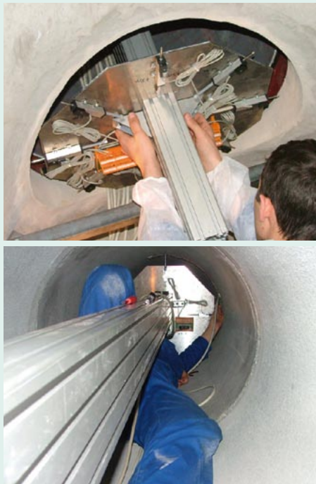
Figure 8: Installation of position transducer assembly above: Installation of a measuring bloc on the measuring bridge below: Positioning of a measuring bloc in the pipe
