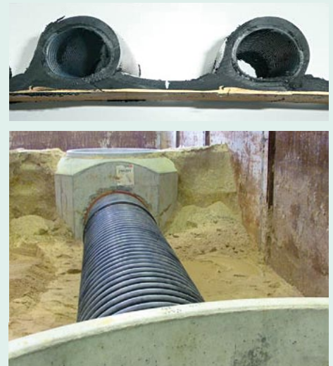
Figure 3: Installation of profiled polyethylene pipes, structure of pipe wall
