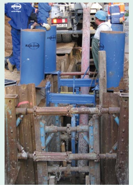
Figure 10 Examples for buoyancy safeguard: Wooden beam construction (above) and RSS® system (below)
