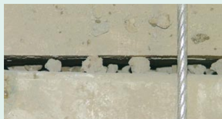
b) Dirt of a gaping joint in the sole area
