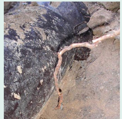
Figure 3 Roots in pipeline trench: root has grown into the sewer and in the end in weakly compacted gore area
