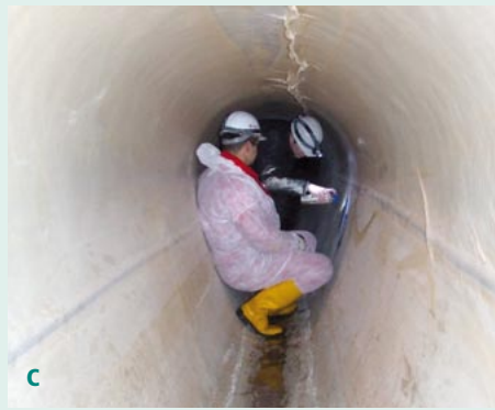
Execution of laser scanning in the sewer
