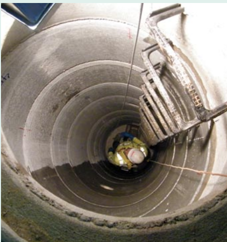
Manhole rehabilitation:
