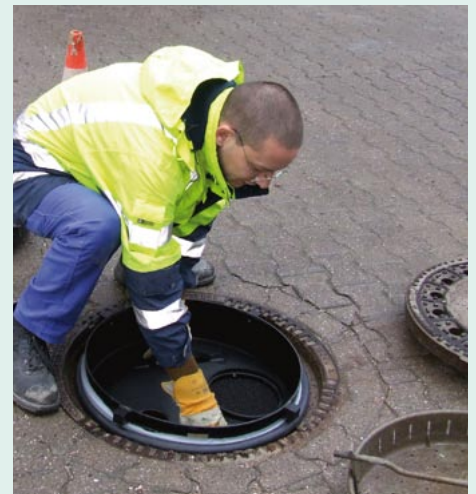
In the practice test: A technician installs odour-filters in manholes on the IKT compound
