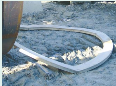
a) Improper support of the pressure transmission devices
