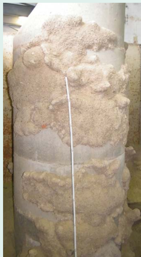
Polyurethane injection body on the exterior of a manhole
