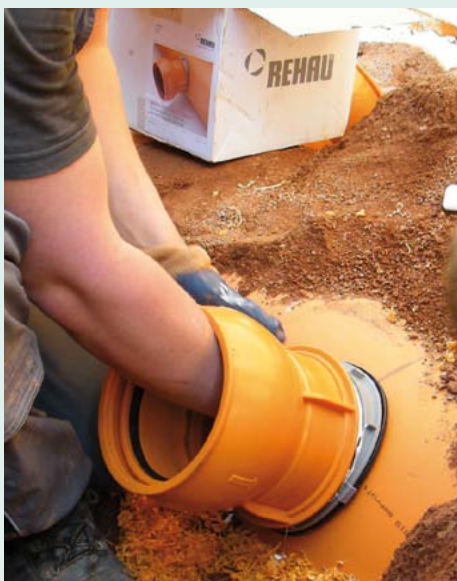
Installation of the Awadock Polymer Connect
