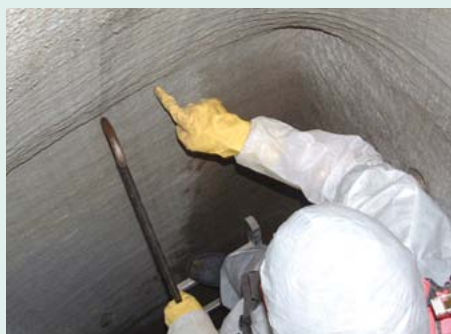
Acceptance inspection: visual assessment of the coating
