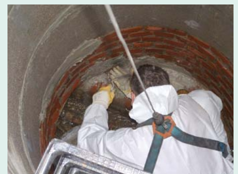
Sealing work in practice: cementitious waterproof plug-compound
