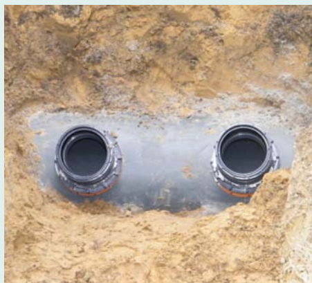
Connex connection following installation (from site study)
