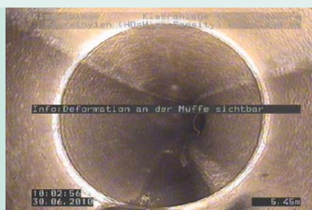
Ovality caused by point load in an HDPE pressure waste-water conduit (photo: Emmerich/Rhine municipal services)
