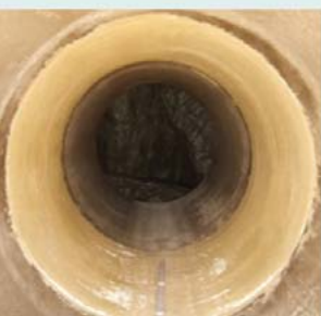
Typical weaknesses: points of material change and/or size transition
