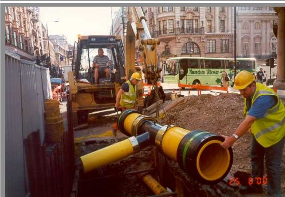
Installing a Tee
