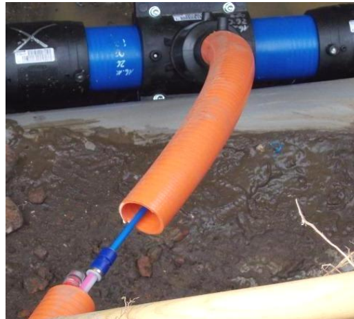
Interface pipe/duct: In the trench
