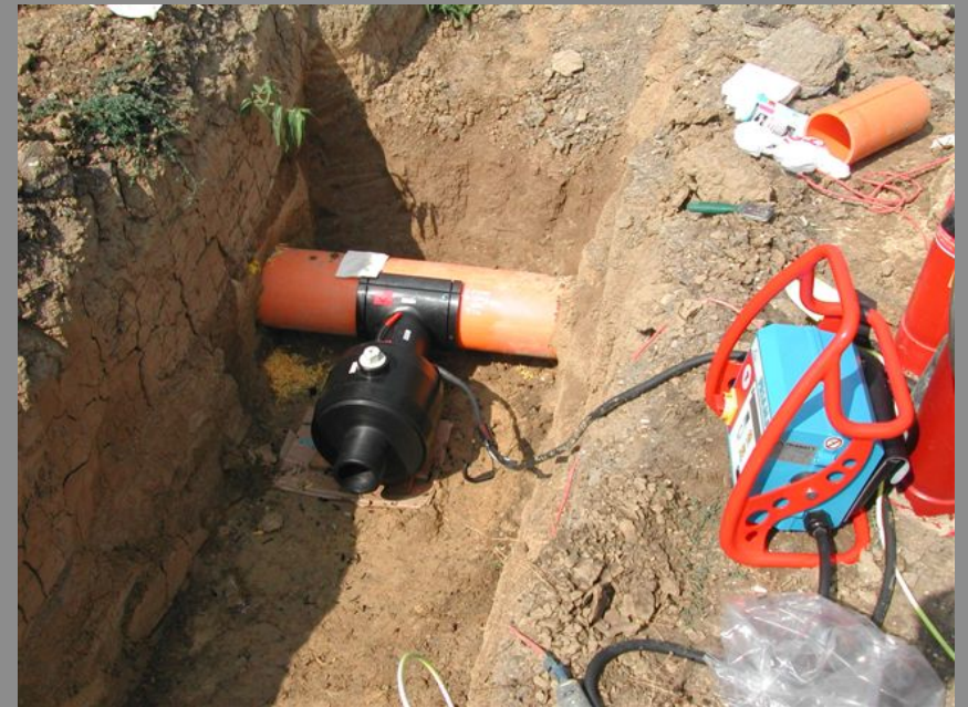
Installing a spigot saddle
