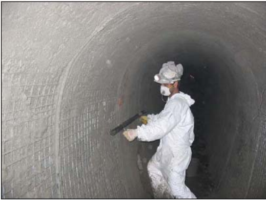
Lining of the brickwork with shotcrete
