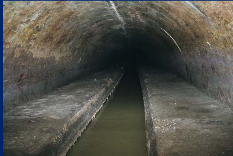
Inside view Sewer
