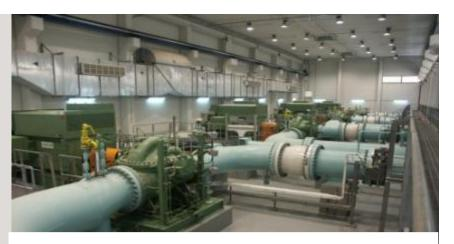
Pipeline System Length: 2 x 180 km Diameter: 64 inch (ca. 1.63 m) Pressure: MOP 56 barg Capacity: 18.900m<sup>3</sup>/h
