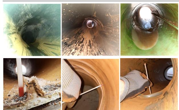
Figure 31. "Wrinkles/obstacles": no conspicuous features with "Compact Pipe" (top left) and "egeLiner" (top centre); longitudinal fold > 6 mm in "Esders HPS Liner" (top right) and "SaniPipe" (bottom left); folds > 6 mm in "Nordiflow W PE" (bottom centre) and "Starline Structure-S" (bottom right).
