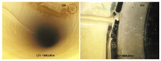
Image 28. Overall visual impression of "SaniPipe": continuous longitudinal fold (left), silicone seal in the fold area at connection 3 (right).
