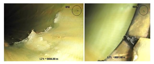
Figure 25. Overall visual impression of "Esders HPS Liner": holes after HP cleaning (left), holes in the rubber of the sleeves after HP cleaning (right).
