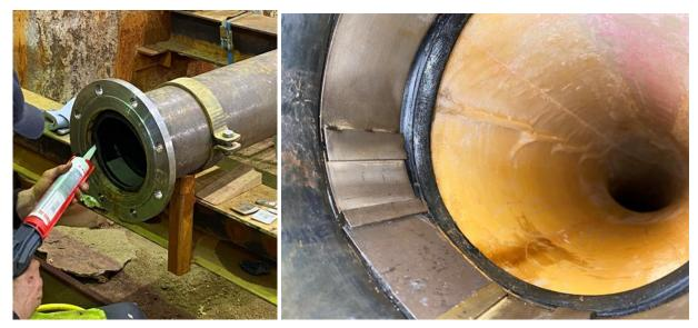
Figure 17. Replacing the sleeves with acetate silicone with "SaniPipe": applying the sealant (left), rework result (right).
