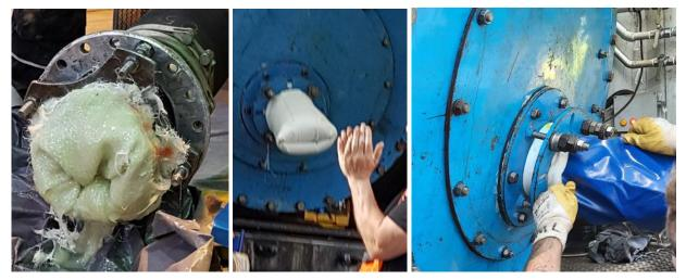
Figure 39 Inversion method: "Starline Structure-S (left), "Nordiflow W PE" (middle/right)
