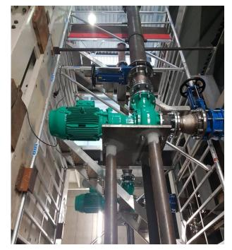
Figure 8. View of the two pumping stations, showing for the nearer pump its support platform, riser pipe with gate valve (leading upwards) and suction pipe coming from the right, also with a gate valve.
