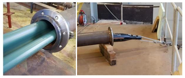
Figure 37. Close-fit insertion process: "Compact Pipe" (left) and "egeLiner" (right).
