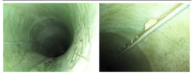
Figure 23. Overall visual impression "Esders HPS Liner": continuous longitudinal fold (left), deposits on continuous longitudinal fold (right).
