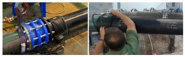
Figure 40. PE flange/ electrofusion couplers: "egeLiner" (left) and "Compact Pipe" (right).
