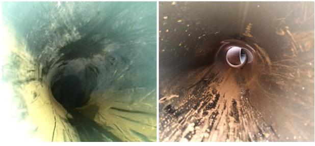
Figure 22. Overall visual impression: Compact Pipe without conspicuous anomalies (left), egeLiner without conspicuous anomalies (right).
