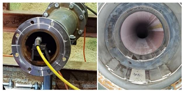
Figure 16. Retightening of the sleeves on "Nordiflow W PE": mechanical device for retightening (left), rework result (right).
