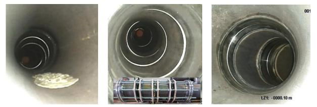
*Figure 32. Damage scenarios "incrustation" (left), "transverse crack with angulation" (centre) and "max. rehabilitable bend" (right).*
